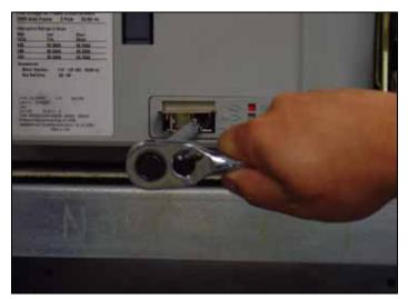
Figure 33.Levering and Position Indication.
